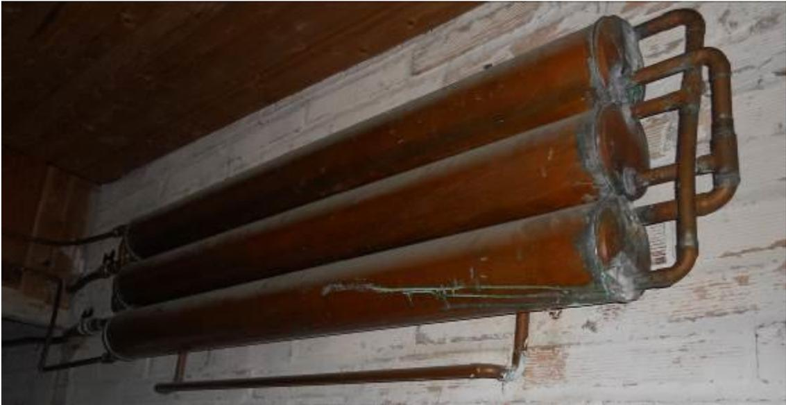
Coil of pipe for heating water
